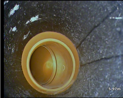
Observation [6]: offset joint 10mm
